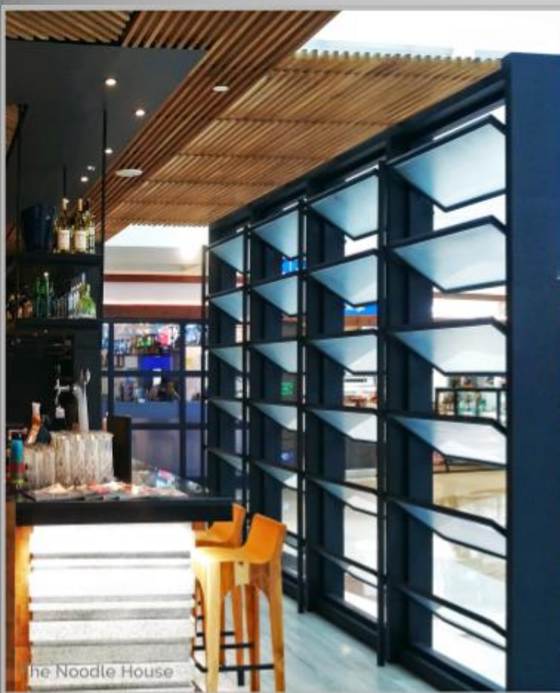
Rotating (awning type) window of create identity and privacy of the store entrance
