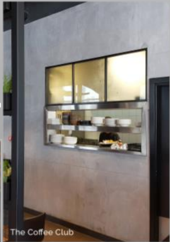
Pass through kitchen window in stainless steel with heating shelf, top glass and metal fixed glass for daylight purpose.
